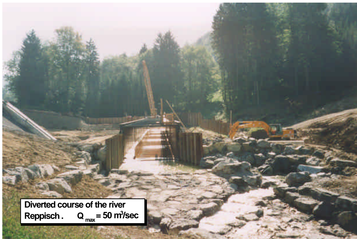
Fig. 20: Diverted course of the river Reppisch in the new bed
