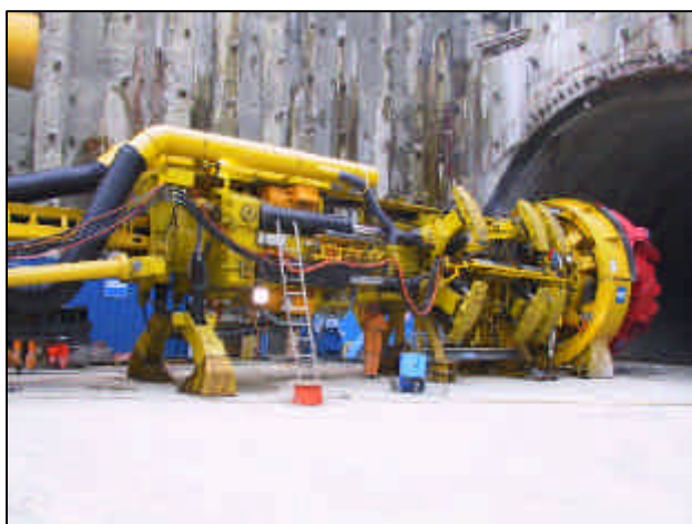
Pilot-TBM with gripper plates in front of portal in Landikon
