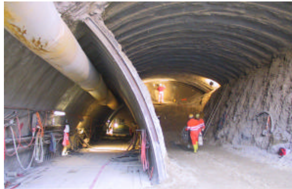
Core boring with steel installation
